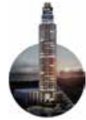
The Regent Under construction.
